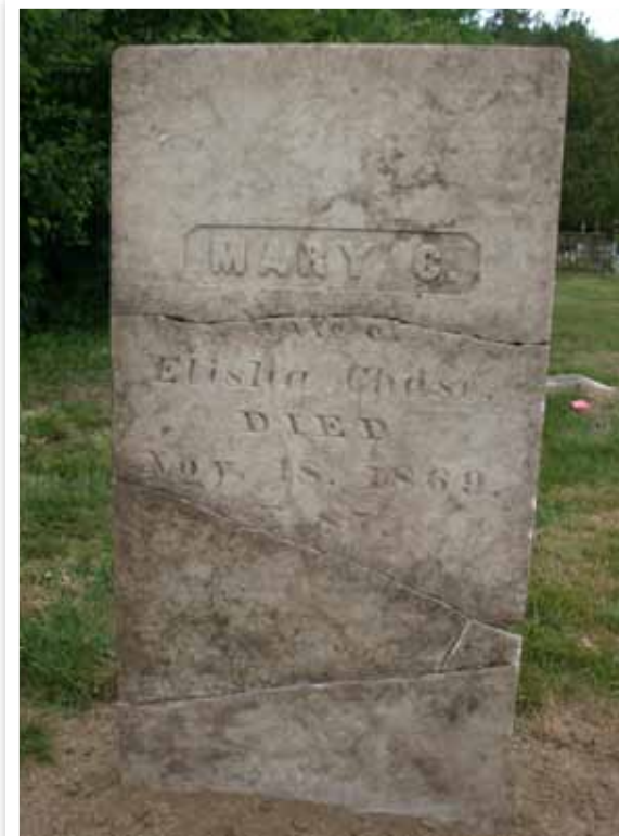
Same stone assembled and upright on a new base
