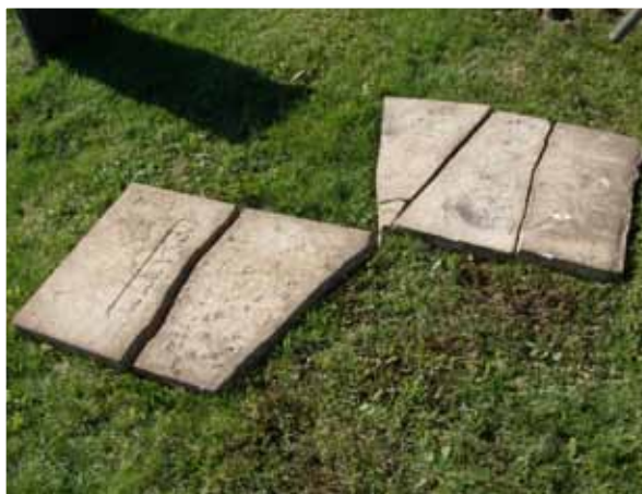
Same stone dug up, cleaned, and prepared to epoxy together
