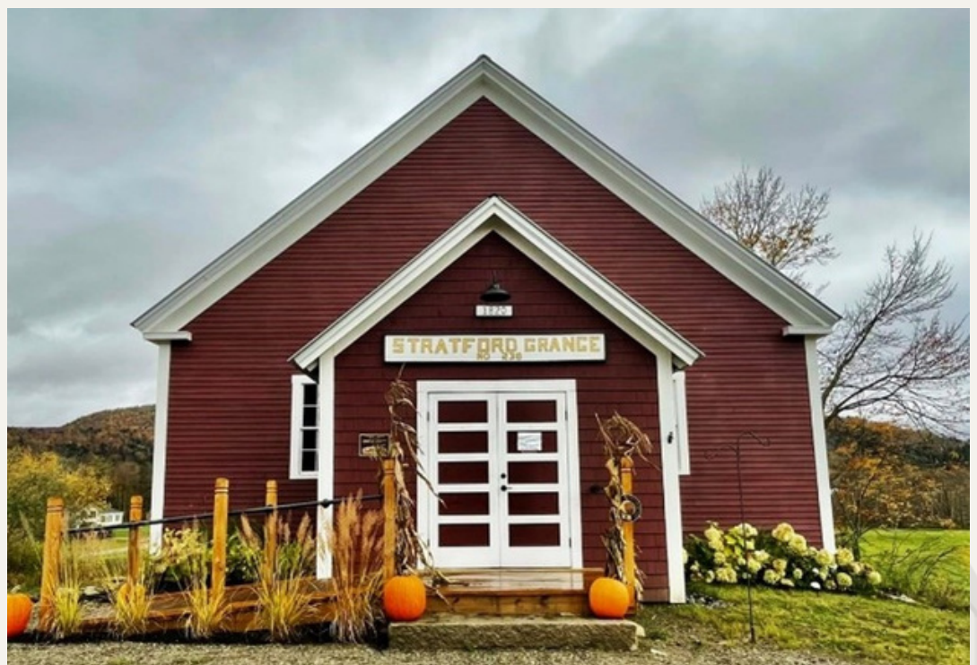
The Stratford Grange after it was moved back from the highway and refurbished (October 2023)
